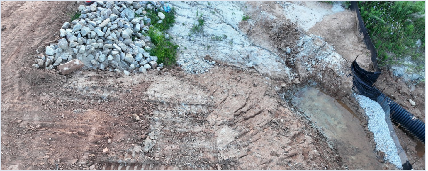
Fig. 6 — Rip-rap apron and outlet protection as installed, at low altitude.
