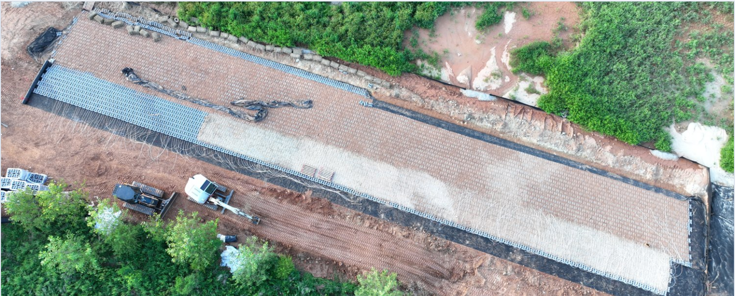
Fig. 3 — Wall and structure placement; alignment and backfill state at capture.
