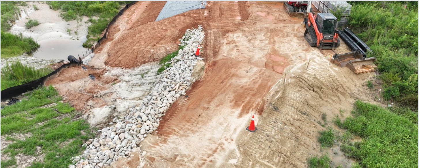
Fig. 5 — Headwall and inlet structure with surrounding grade, before cover.
