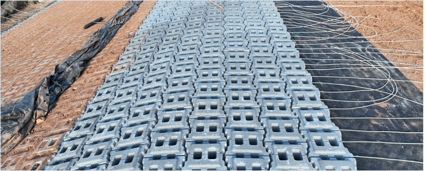
Fig. 4 — Geogrid and base placement, photographed from directly overhead prior to cover.
