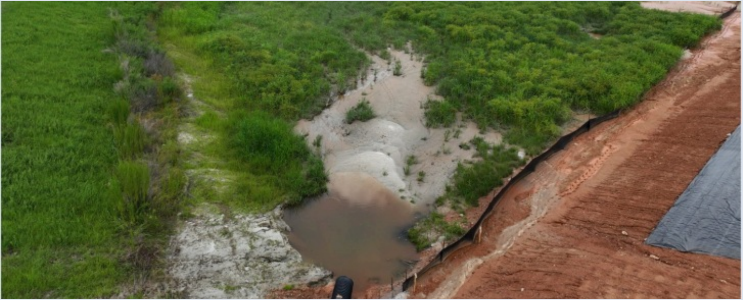
Fig. 8 — Sediment basin. Water level, vegetation establishment and berm condition after weather.
