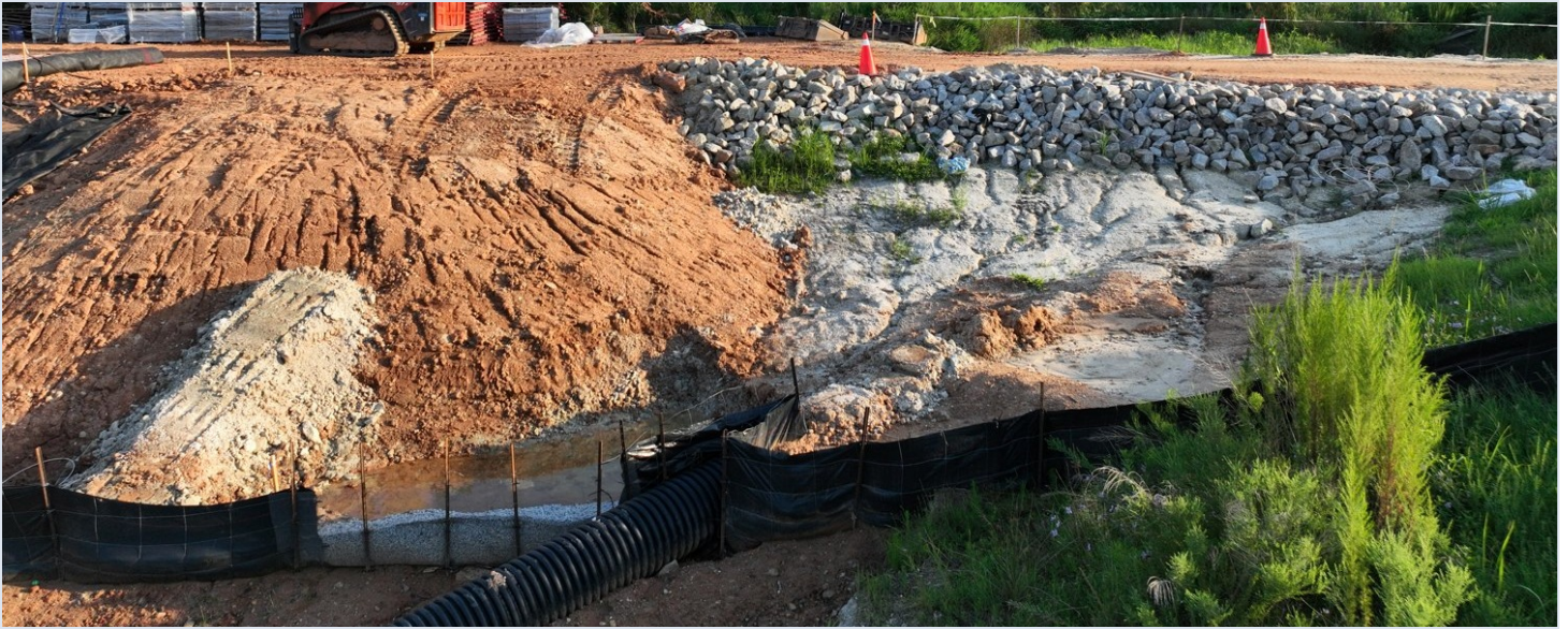
Fig. 2 — Material stockpile and equipment staging on the date of flight.
