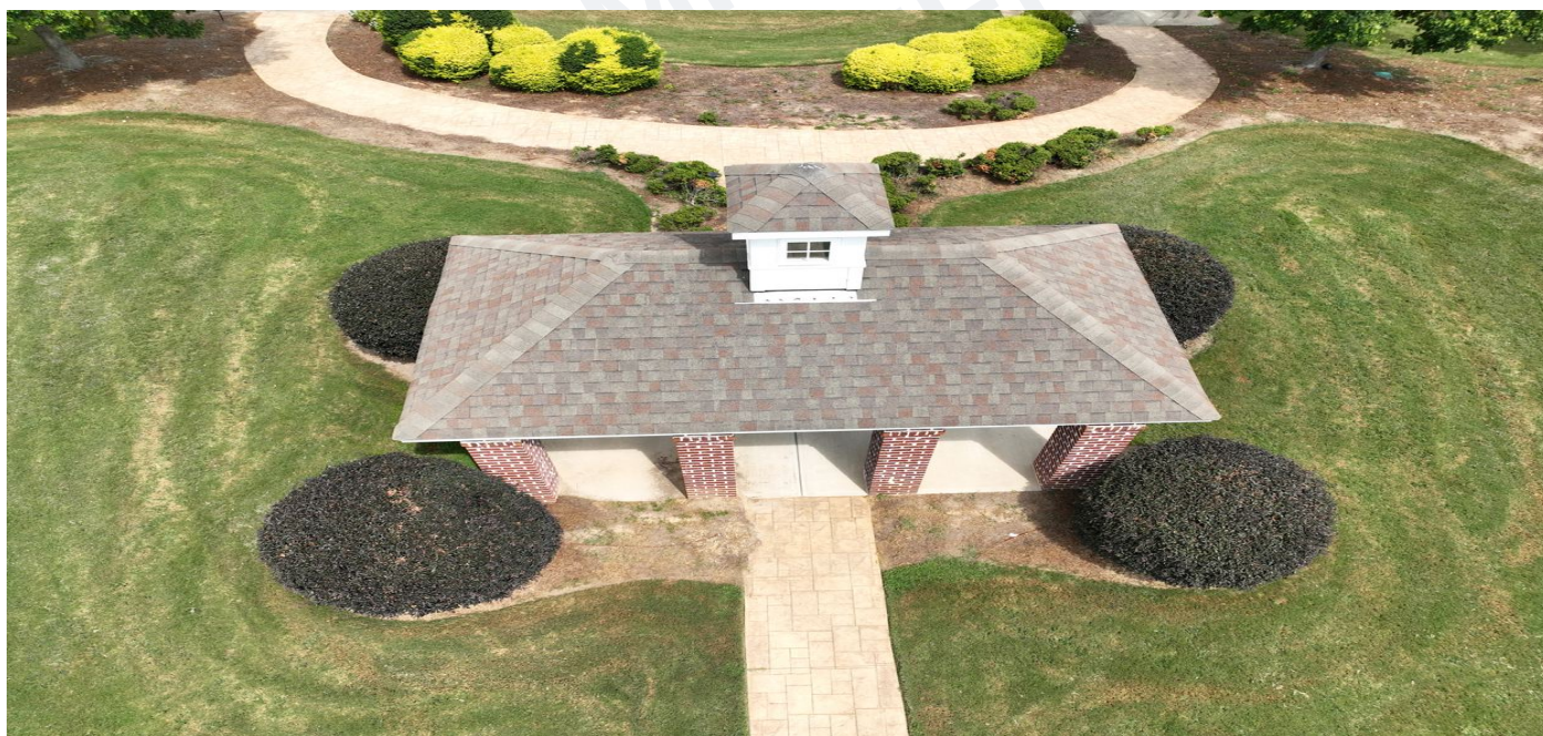
Fig. 4 — Picnic pavilion from directly overhead. Every plane, hip and the cupola in one frame — the view a ladder cannot give — with the walkway and bed edging around it.
