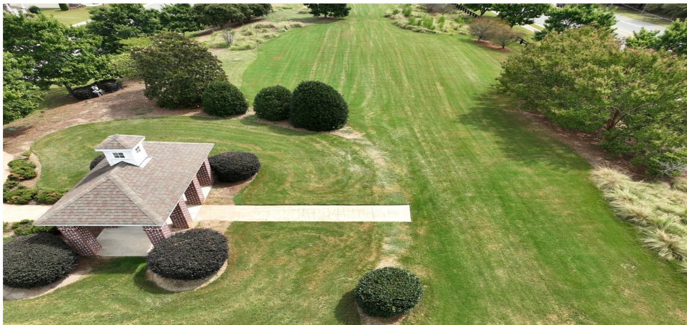
Fig. 5 — Pavilion at elevation with the common lawn behind it. Roof, brick piers and open bays as found, and the walkway running out into the maintained area.
