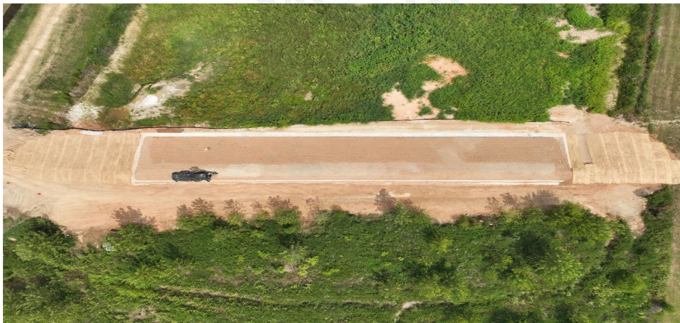
Fig. 8 — Active work area. Permeable paver pad placed with the perimeter curb formed, silt fence along the wooded edge, and straw stabilization begun on the graded slope.
