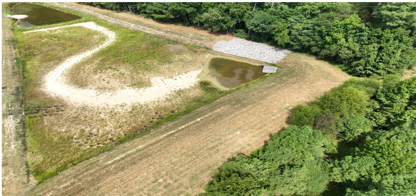
Fig. 7 — Stormwater control measures. Sediment accumulation and established vegetation across the forebay, the lower basin holding water, the outlet structure clear and the riprap outfall in place.
